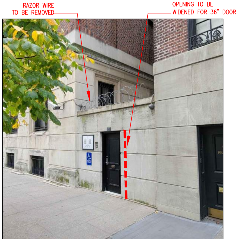
DOOR TO REAR COURT ON 69TH STREET
