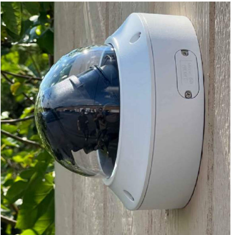
DETAIL OF PROPOSED CAMERA WITH HIDDEN CONDUIT
